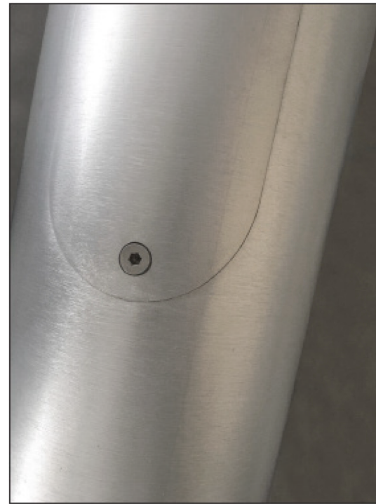
FLUSH HATCH DETAIL
